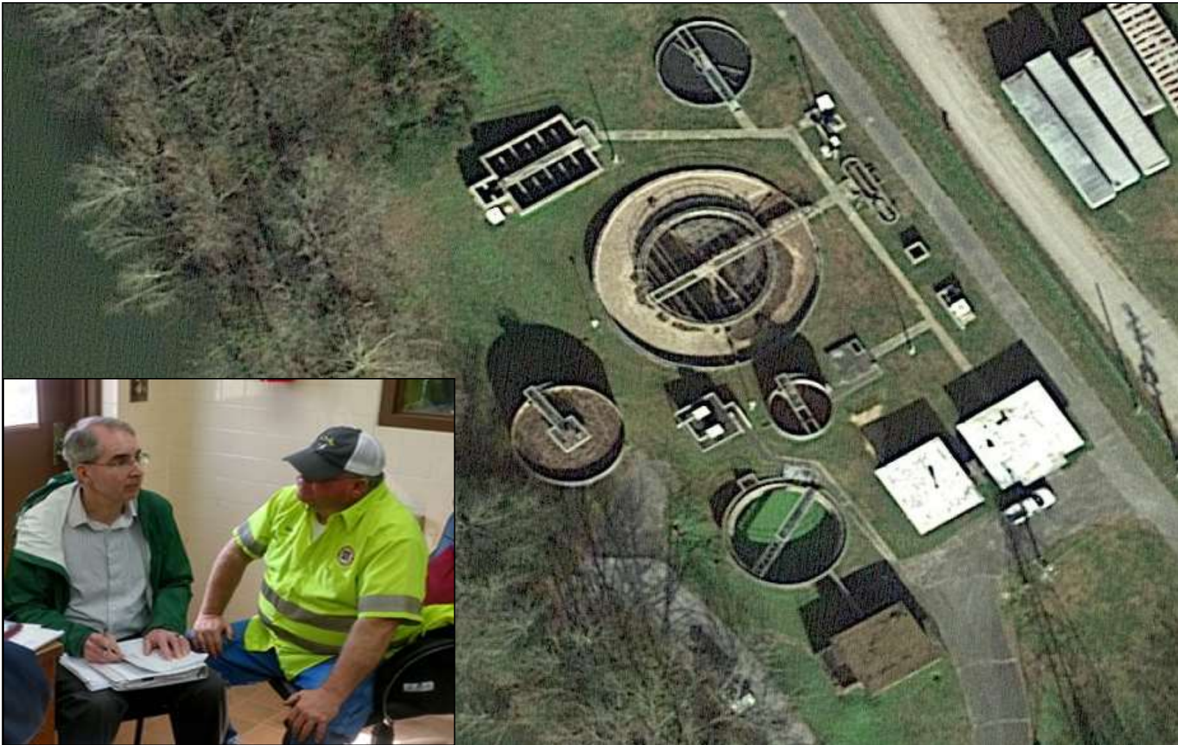
Carthage Wastewater Treatment Plant
